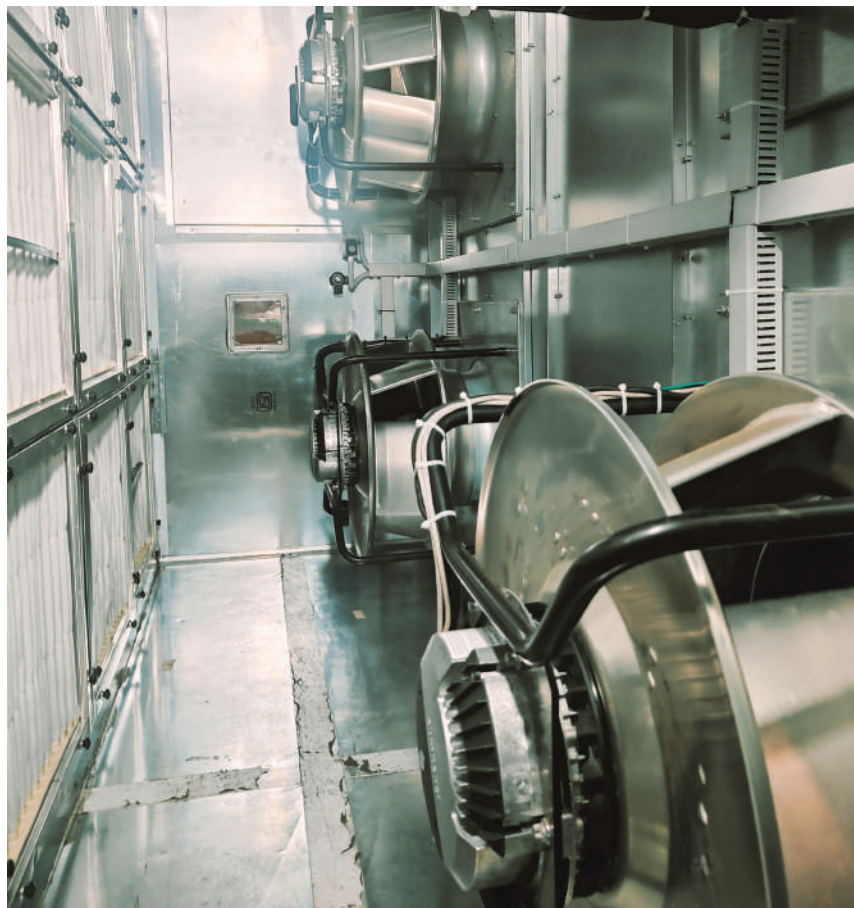
EC fan installation at AHU
