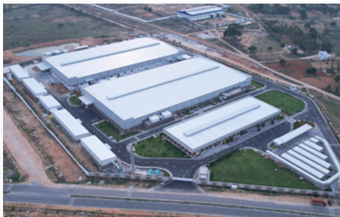
Manufacturing plant at K R Pete, Mysore
