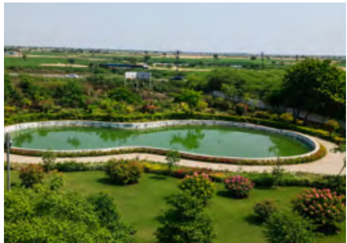
Water Conservation at Sanand Plant
