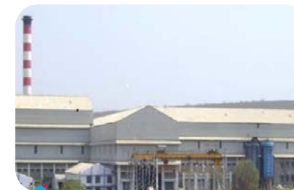
Sugar and Co-generation Factory Ramdurg – Karnataka
