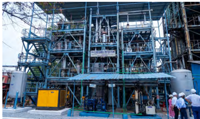
Coal Gasification Pilot Plant facility, capacity; 0.25 TPD, IICT Campus, Hyderabad
