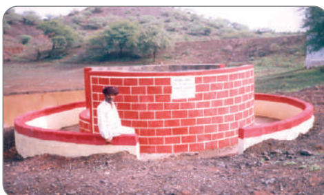
Construction of Wells
